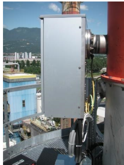
Sampling unit installation
